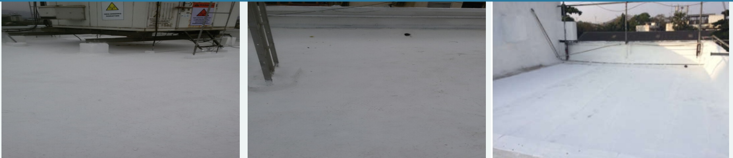
Terraces coated with Flexi-Crete PM 650
