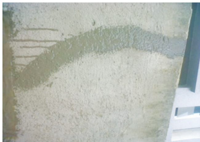
Crack Repaired Using Flexi-Crete SC300
