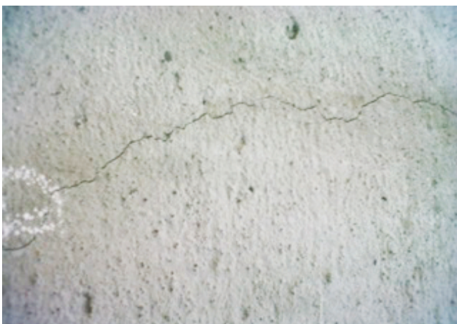
Before Crack Repair
